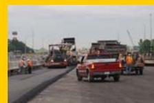
*ITCPs control the movement of vehicles and equipment inside the work zone. Well constructed ITCPs are intended to limit exposure of WOF to vehicles and equipment.*
