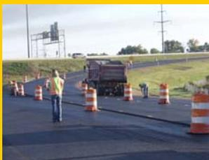
*In the U.S. highway construction industry an average of 22 fatalities occur each year from collisions between construction equipment and a worker. Half of all the backing fatalities involve a dump truck.*
